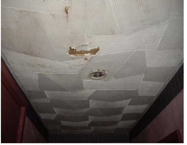
Artex Textured Coating to ceiling
